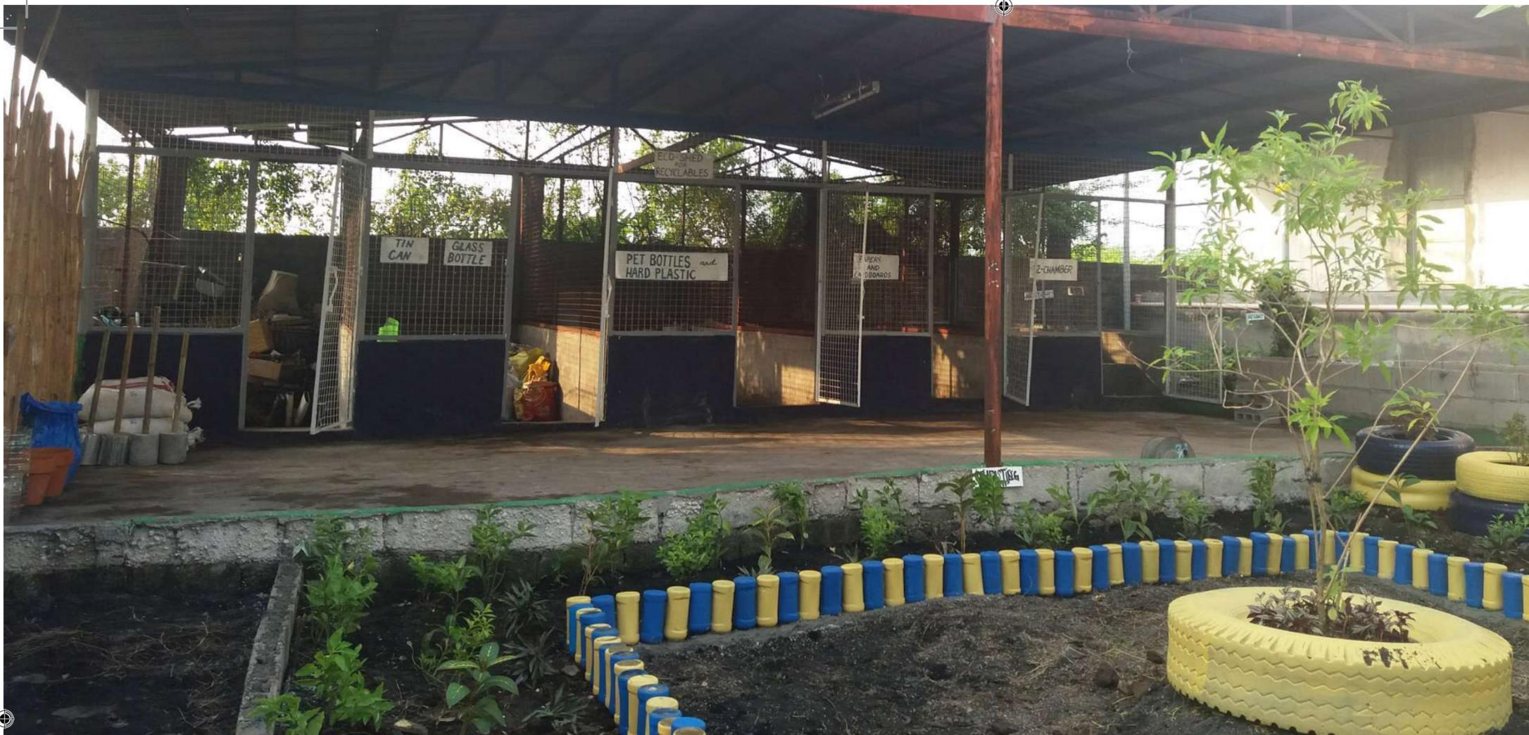
A materials recovery facility (MRF) in Malabon City. Functioning MRFs have composting areas for biodegradables and temporary storage rooms for recyclables.
